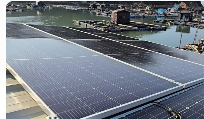
20MW Ground-mounted PV Station in the USA
