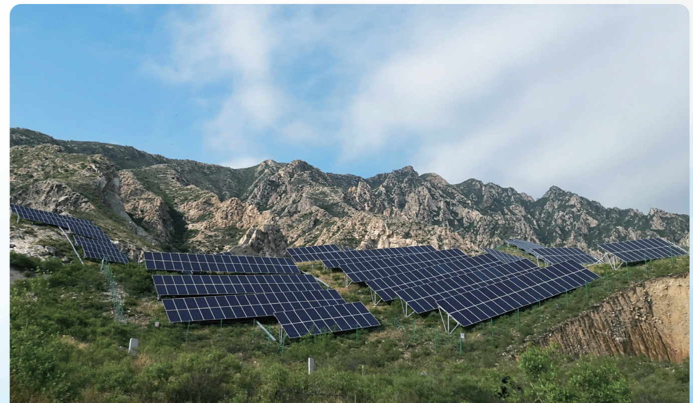
500MW in Zhangjiakou
