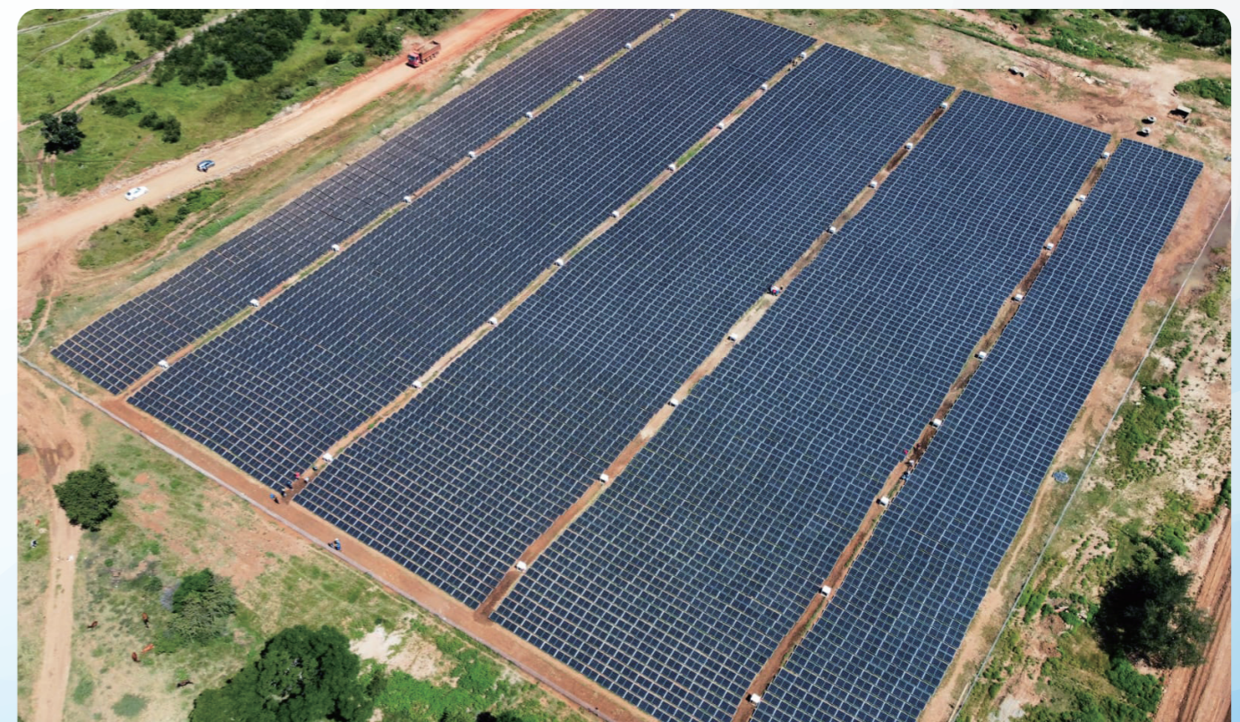
PV project of gold mine in Zimbabwe
