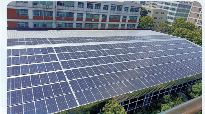
200KW PV Project in Jialong Paper Industry
