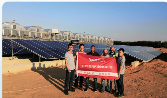
PV Project in Jeddah, Saudi Arabia
